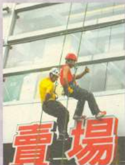
來自萬多尼亞的攀岩大師正沿著家樂福外牆垂降而下。 Taiwan's best rock climbing expert rappelled along the outside wall of the Carrefour Ta Zhi store.
